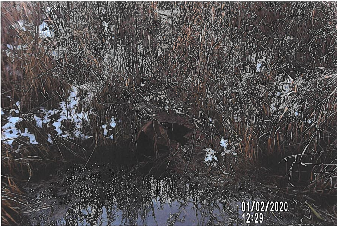
PICT# 2617 IS LOOKING SW SHOWING 30" CMP OUT LET ON NWSIDE OF RR ACCESS DRIVE ON NE SIDE OF DRAINAGE STRUCTURE WITH END CMP ALL MANGLED UP BUT FLOWING WATER LEVEL AT 20"
